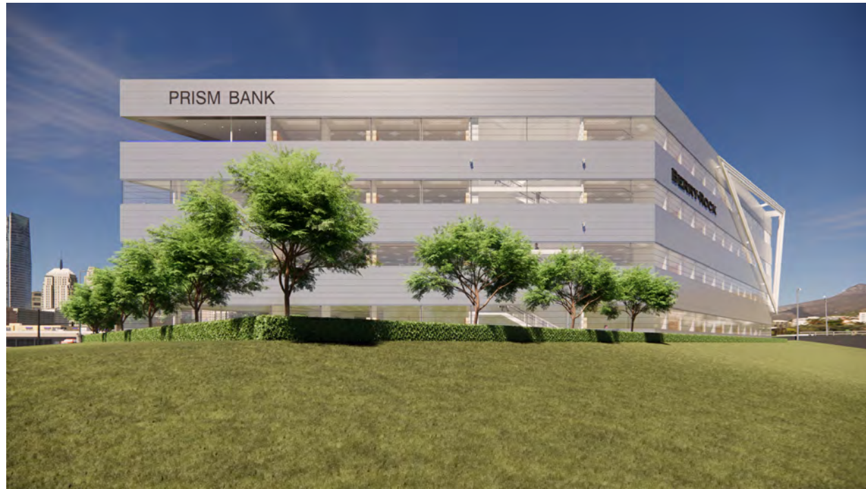
1. VIEW LOOKING EAST FROM ON RAMP
