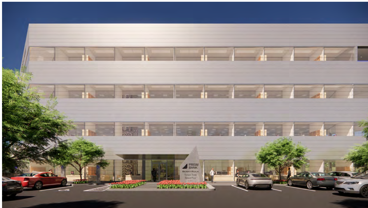
3. VIEW OF MAIN ENTRY
