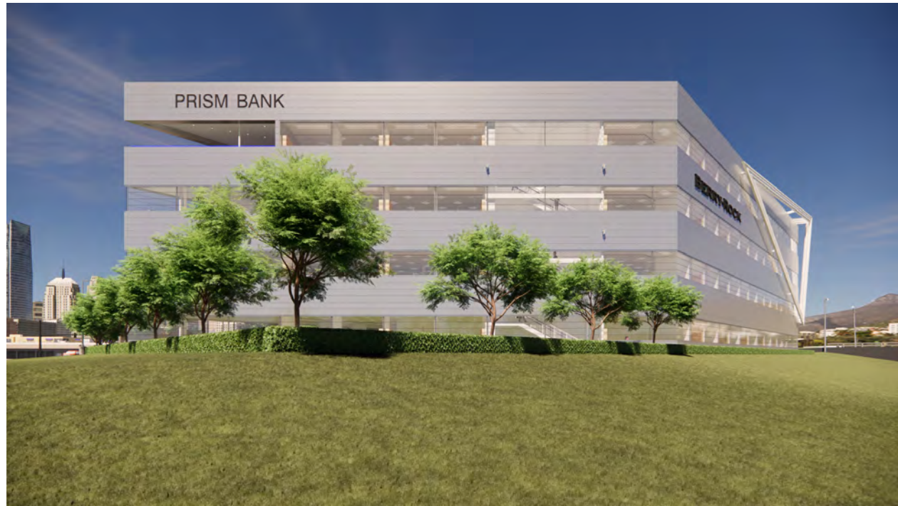
1. VIEW LOOKING EAST FROM ON RAMP
