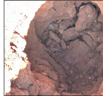
DOWN HOLE PHOTO OF UTILITY DATE: 08-09-2023
